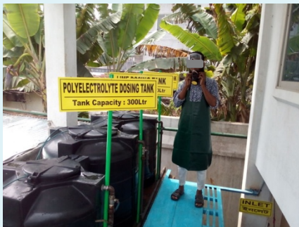
Improved Health & Safety: PPE being used on ETP
