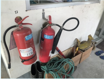
Improvement of fire safety: Installation of fire fighting equipment
